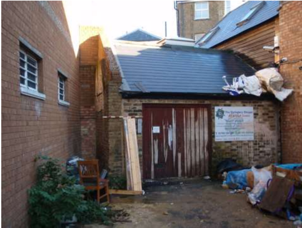
Plate 4. View of south entrance to the building from Leslie Smith Drive showing on the left an earlier phase of construction in yellow stock bricks with a modern rebuilt south wall in reused bricks butting to the yellow stocks. Sloping roof laid with modern slate tiles to a modern flat roof pierced by modern plastic square fanlights.
