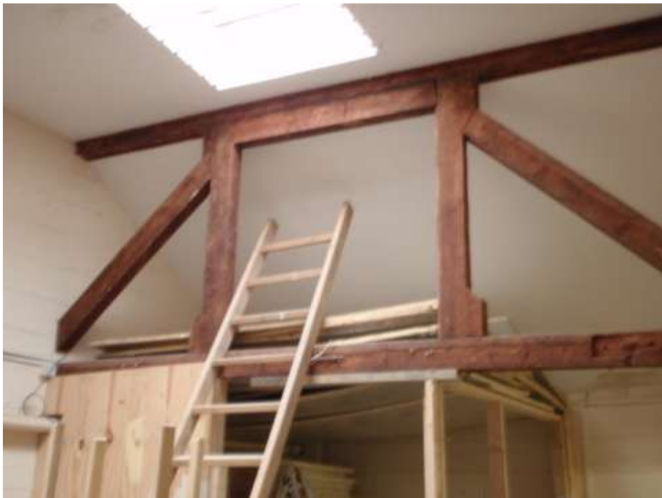
Plate 5. View of interior of south building showing reused radial machine cut Queen Post roof truss and purlins topped by a reused radial machine cut timber joist to facilitate construction of the modern flat roof. The west wall (left) is of modern concrete block construction as is the wall to the north.
