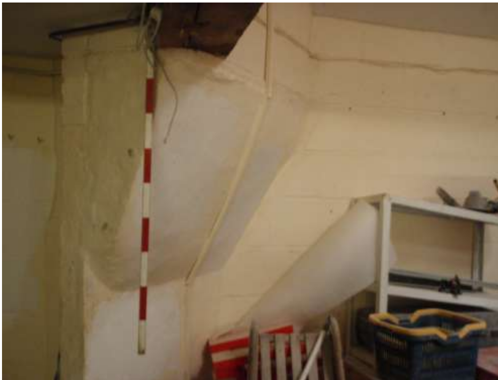
Plate 7. View of odd arrangement of cantilevered blockwork to hold up the reused floor beam presumably because the beam was too short.
