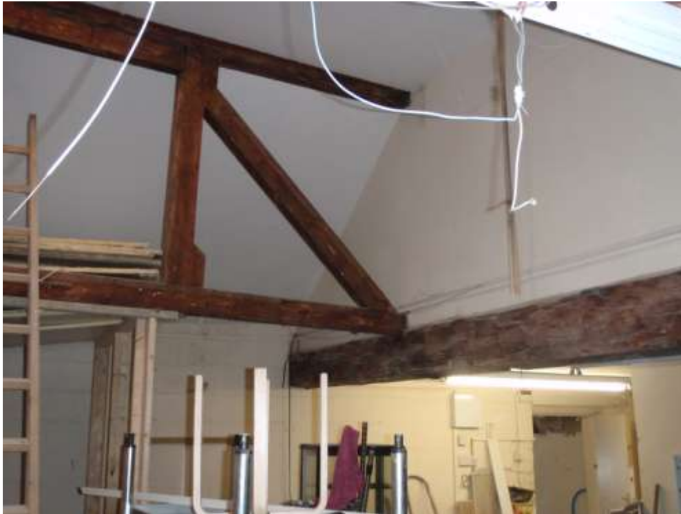
Plate 6. View of interior of south building looking to the east and showing the reused Queen post truss sitting on an reused earlier adzed timber floor beam with modern construction above it.
