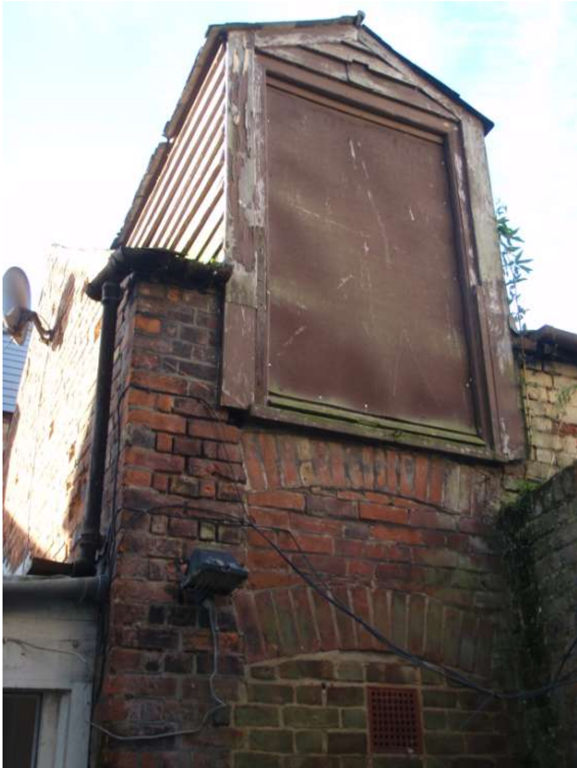
Plate 1. View of north east corner and showing part of the original fabric of mixed orange to dark red brick laid in a type of English bond with buff penny-struck lime mortar. Two segmental arched windows both blocked with later brickwork and above a gabled dormer loading bay of timber construction with feathered edged boarding on the timber stud wall cheeks. To the right can be seen the yellow stock bricks of a later reconstruction.
