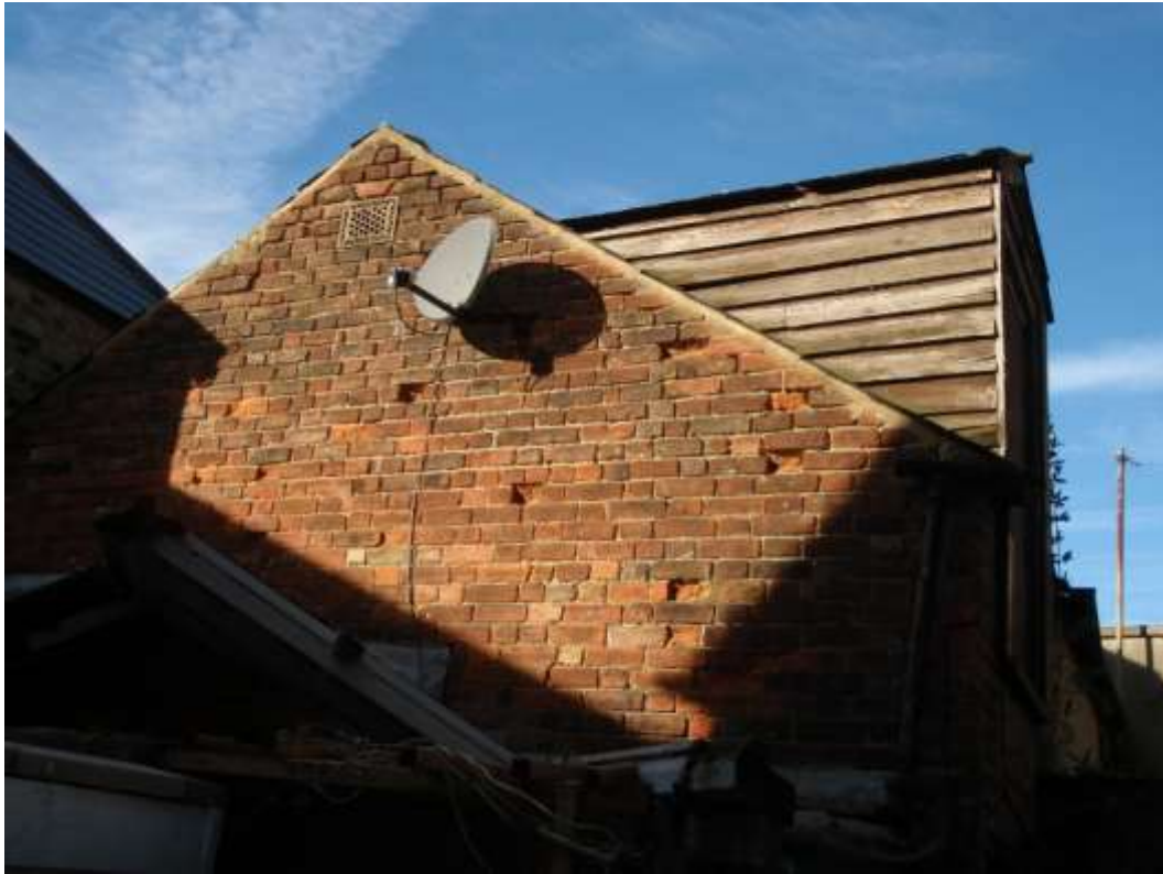
Plate 2. View of east gable showing part of the original fabric of mixed orange to dark red brick laid in a type of English bond with buff penny-struck lime mortar and the cheek face of the timber dormer.
