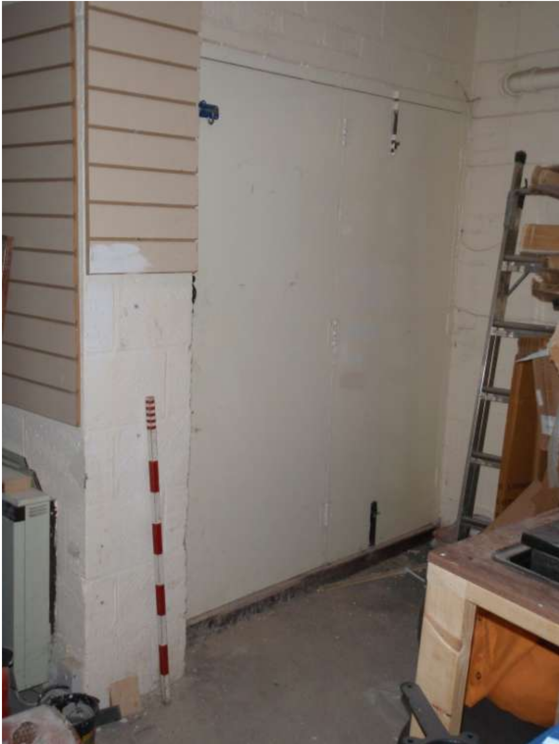
Plate 8. View of interior of north building showing modern concrete floor, modern blockwork and part of the original brick wall on the right.
