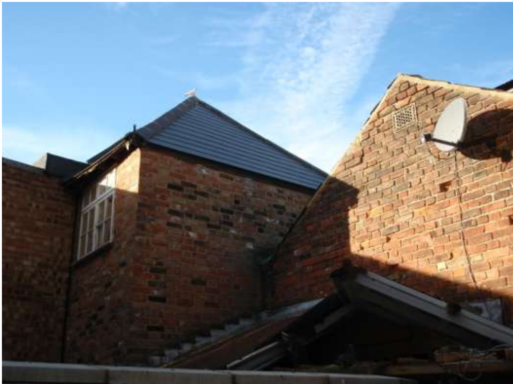
Plate 3. View of east gable showing the new build adjoining building.
